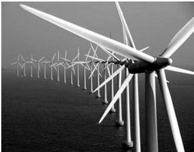
An offshore wind farm off Denmark.
