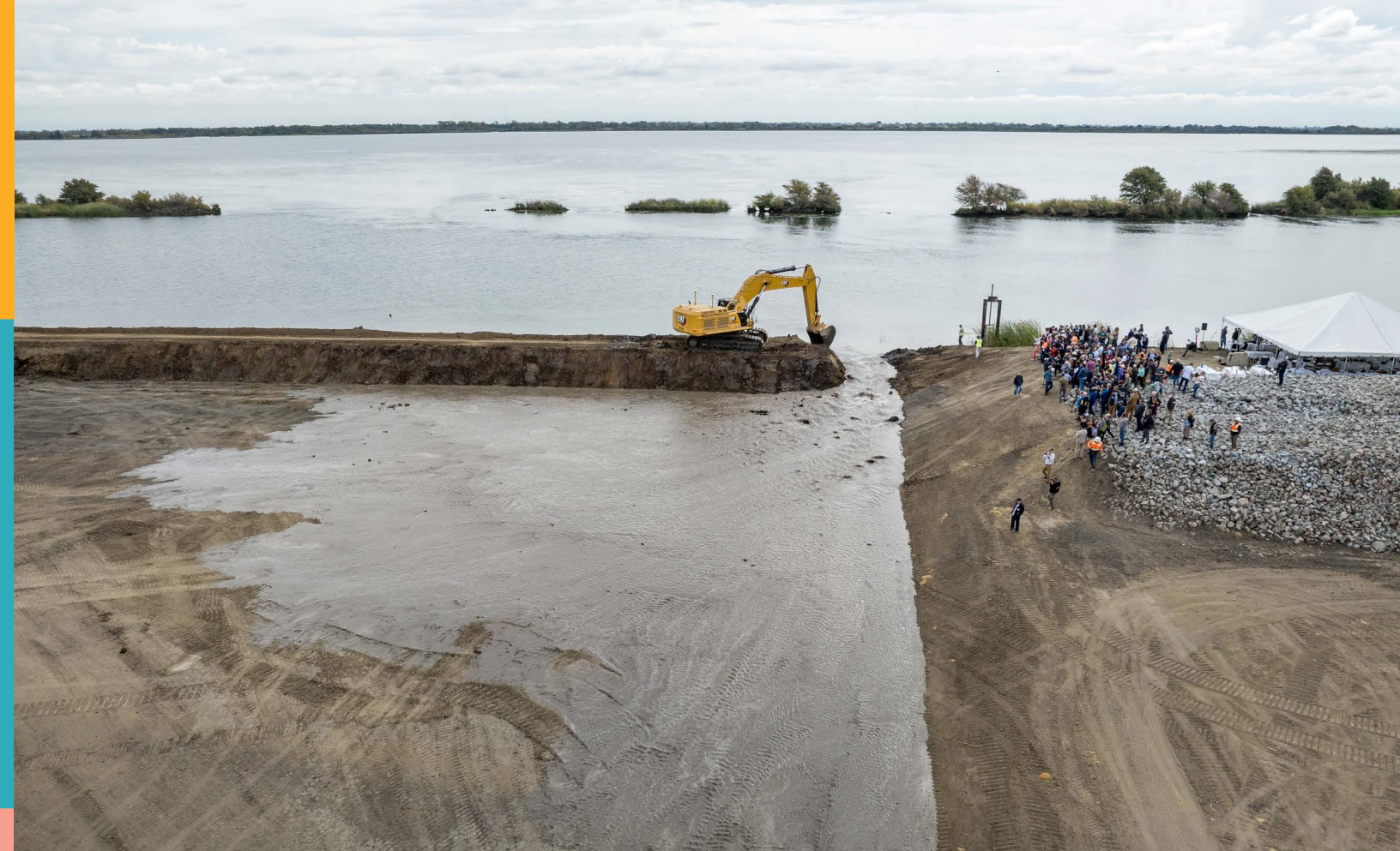
Final notching of the levee at Lookout Slough in Solano County, Credit: DWR
