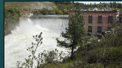
Nine Mile Dam, Avista Corp
