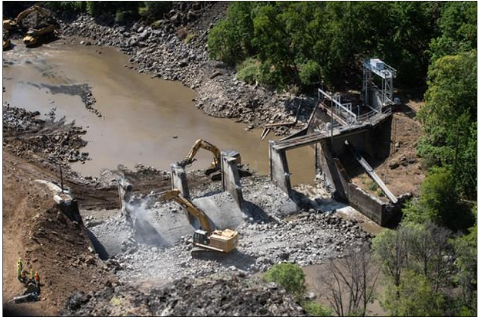
Copco-2 dam removal. Credit: Shane Anderson, Swiftwater Films
