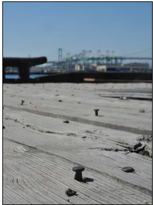
The wood is rotting away leaving the spike nails as dangerous obstacles.
