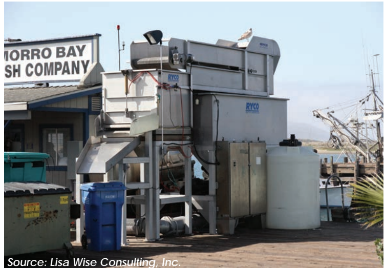
Source: Lisa Wise Consulting, Inc. Newly installed wet fish pump for off loading at Morro Bay Fish Co.
