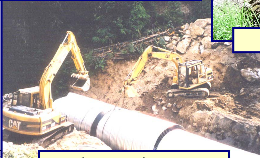
Culvert Replacement
