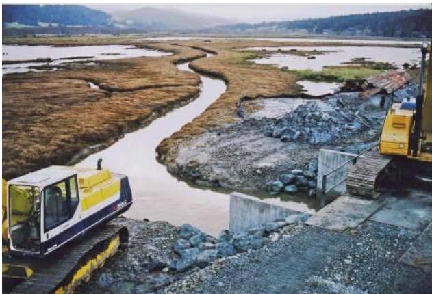
Connection between Hookton Slough and Salmon Creek (Humboldt Bay population) was restored with a new tide gate.
