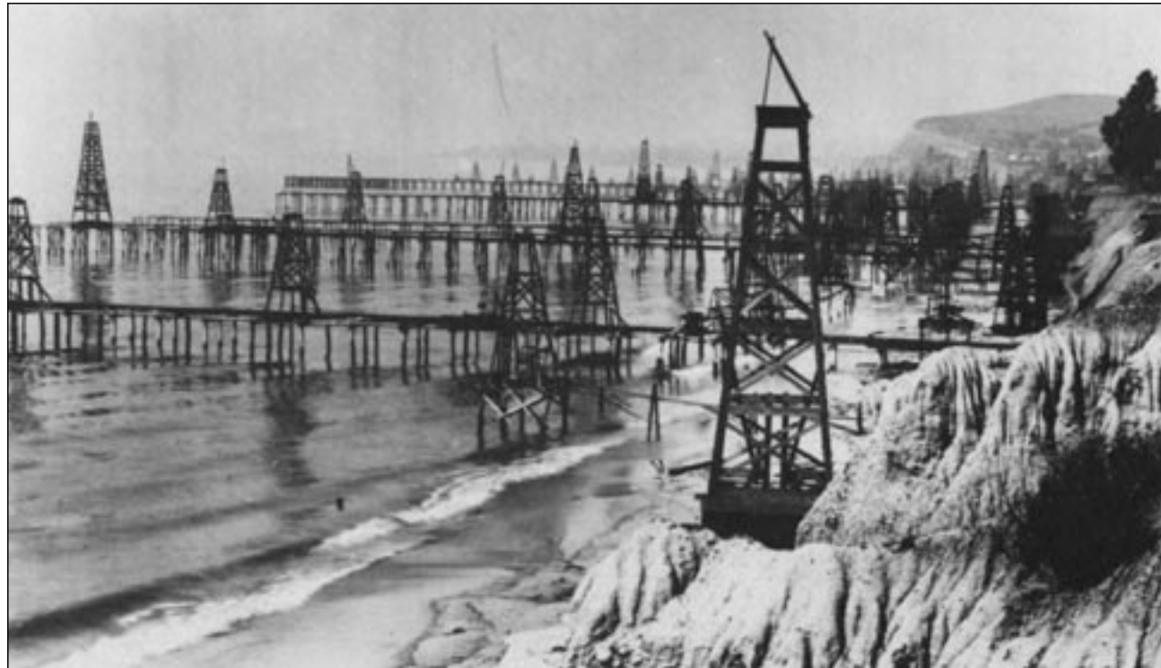
Figure 2.1. Oil piers off Summerland, California, about 1904 (from Rintoul 1990).
