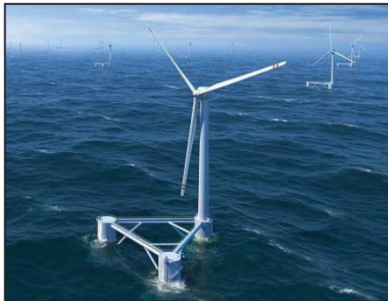
A rendering of Principle Power's WindFloat floating wind turbine - one potential future use of the ocean.
